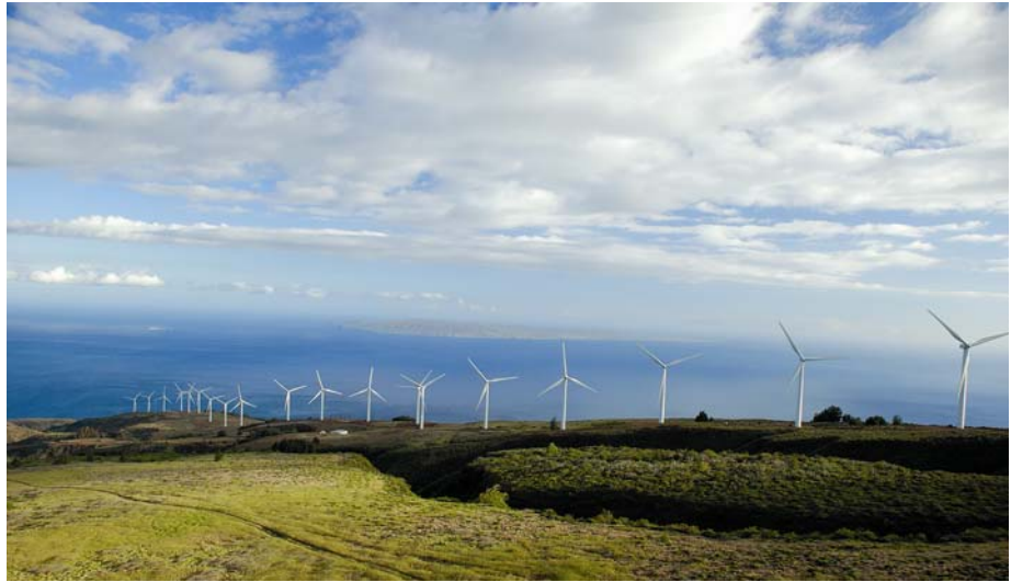
Kaheawa Wind Power turbines in Hawaii. Photo courtesy of UPC Wind.
