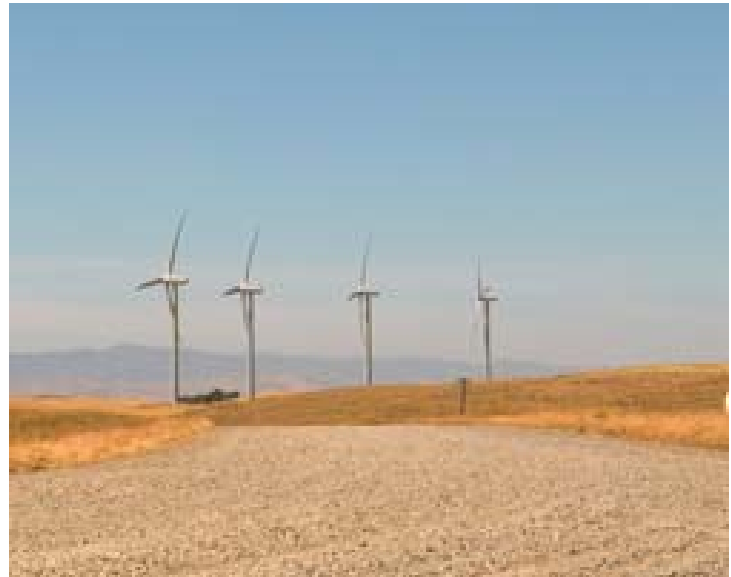
Wind turbines at the Highwinds wind project in California. Photo courtesy of FPL Energy.
