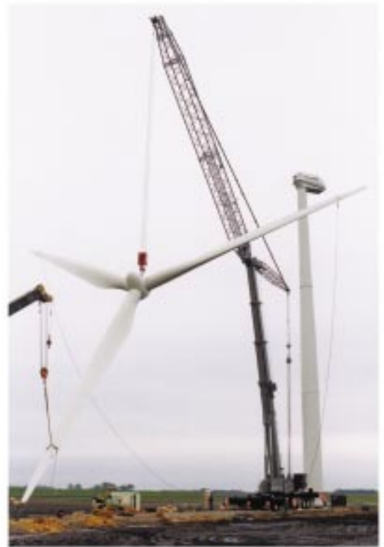
The rotor and hub system weighs 30,800 lbs
