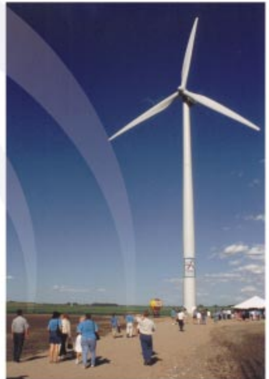
The rotor and hub system weighs 30,800 lbs
