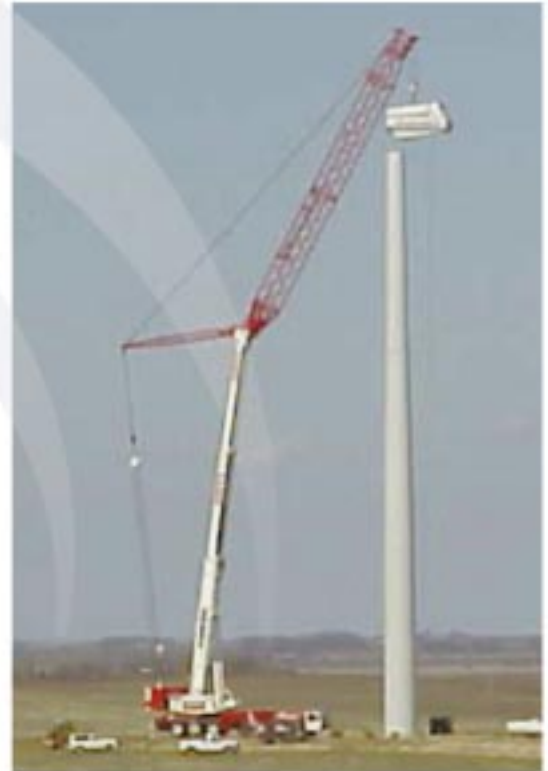
The towers consist of three pieces which are bolted together on the inside
