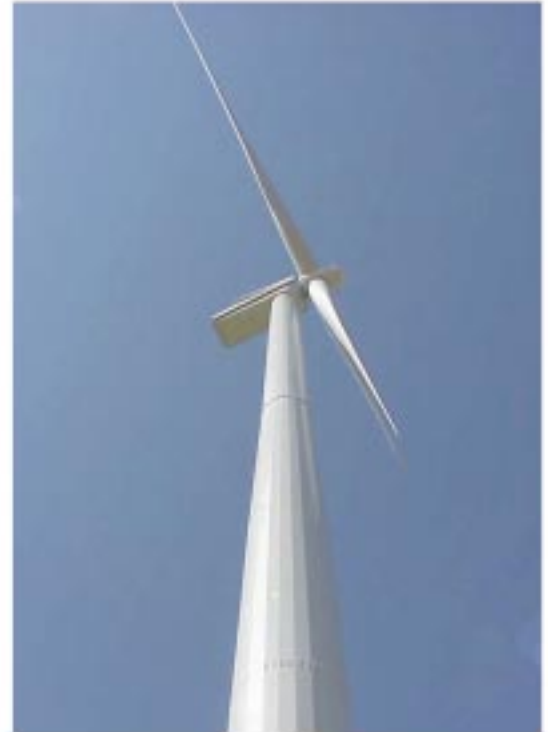
The towers consist of three pieces which are bolted together on the inside
