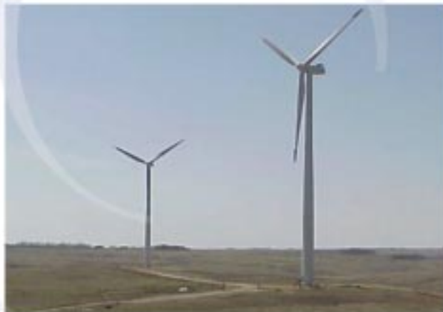
The wind turbines are remote controlled and monitored via fiberoptic cables
